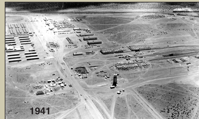
An aerial view of the UMCD under construction. Courtesy of the Library of Congress.
